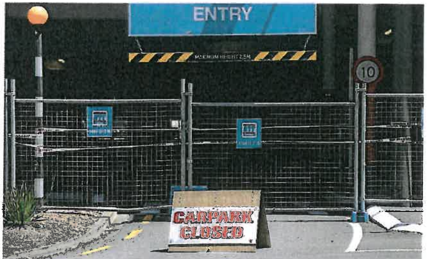
Quarantine in Lower Hutt was damaged and a section of it has been demolished.
